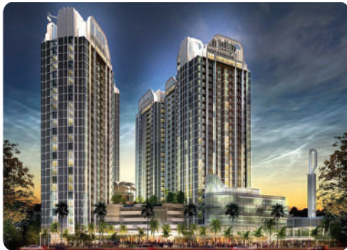
Arandra Residence – cempaka Putih
